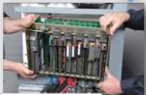
Remove the 1771 chassis from the control cabinet.
